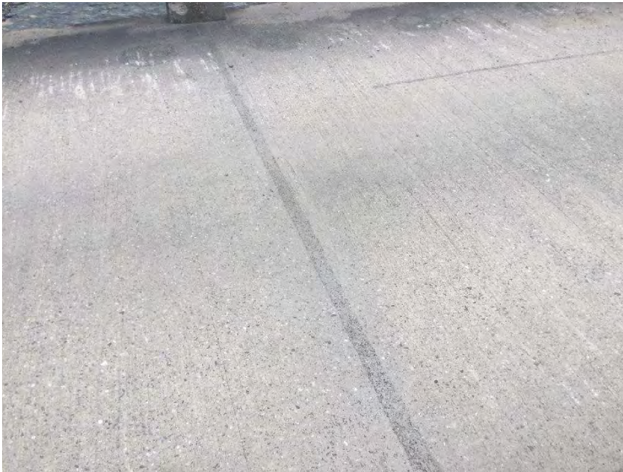
Photo 12 Typical grouted deck panel joint condition
