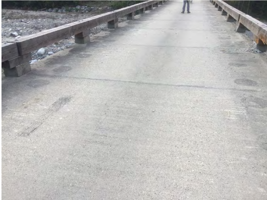
Photo 9 General deck condition
