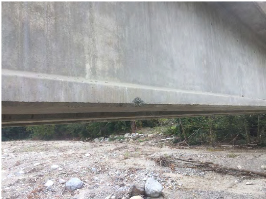
Photo 20 Typical span 2 girder condition
