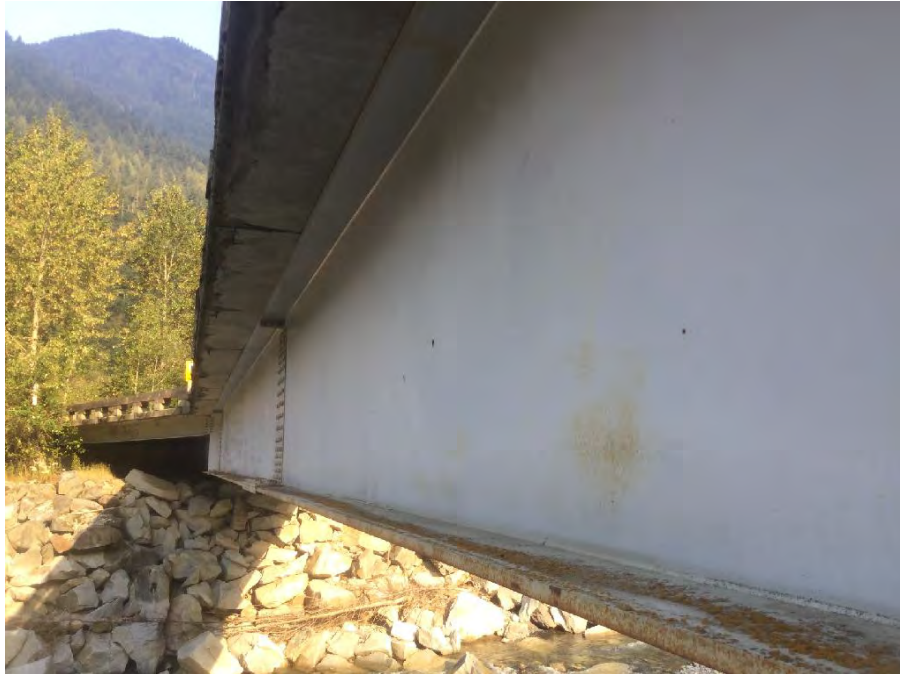
Photo 21 Typical span 3 girder condition
