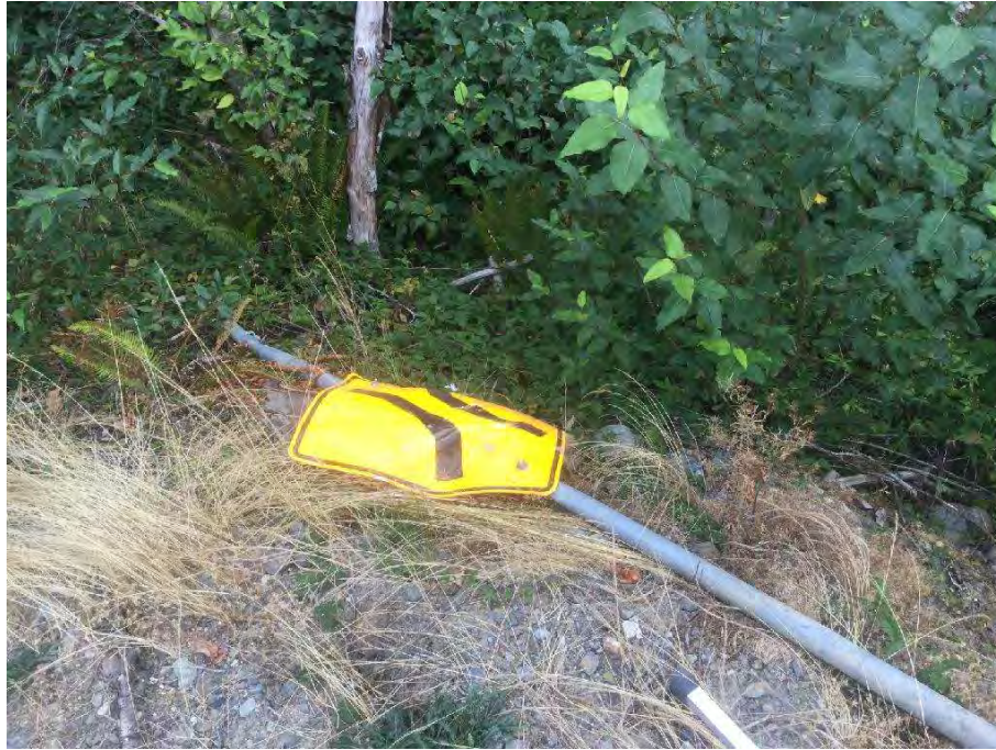
Photo 31 Left 'Narrow Road Ahead' sign knocked over
