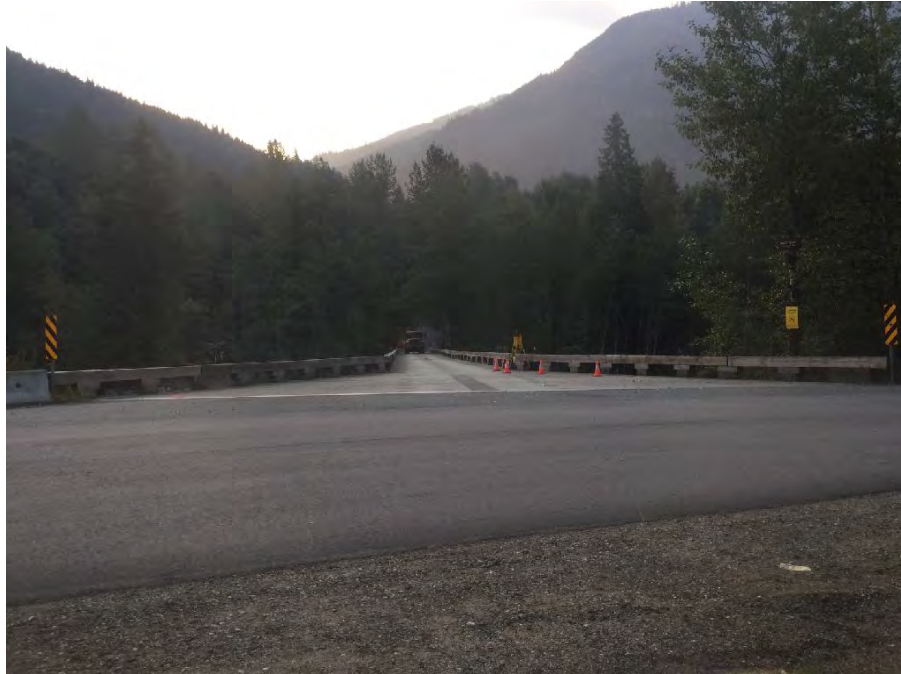
Photo 7 Right approach looking towards bridge
