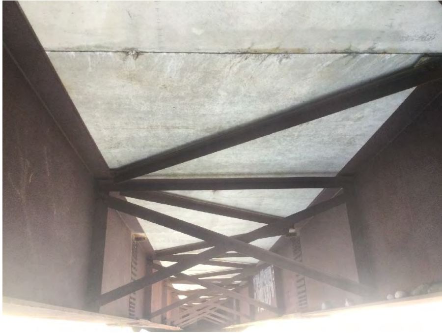
Photo 23 Typical underside of deck condition
