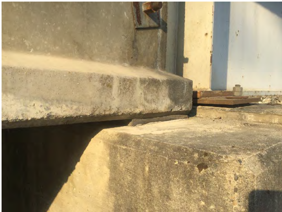
Photo 24 Typical bearing condition
