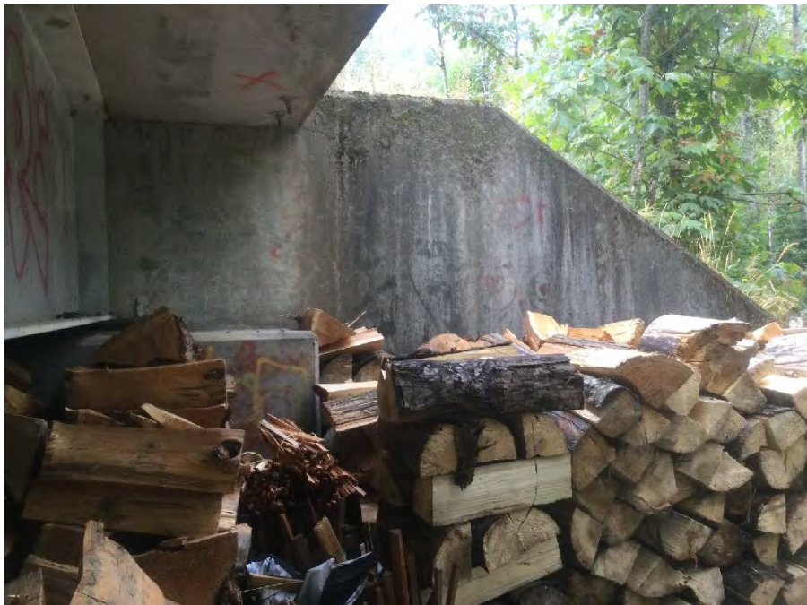
Photo 16 Left downstream wing wall
