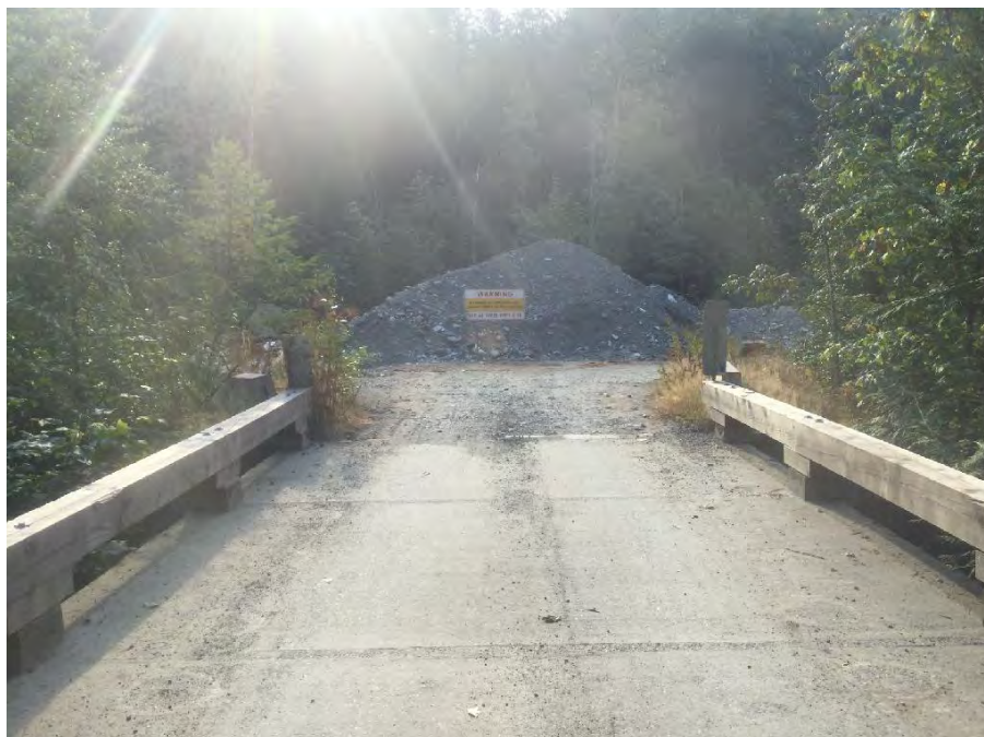
Photo 6 Left approach looking away from bridge
