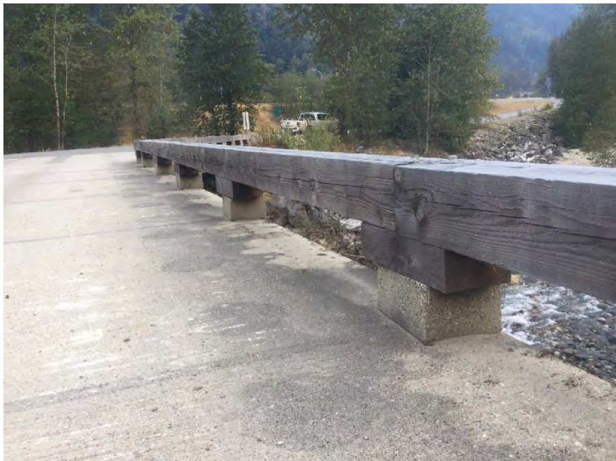
Photo 10 General railing condition
