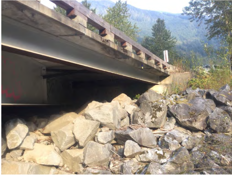
Photo 17 Right upstream wing wall
