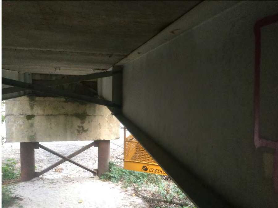
Photo 19 Typical span 1 girder condition
