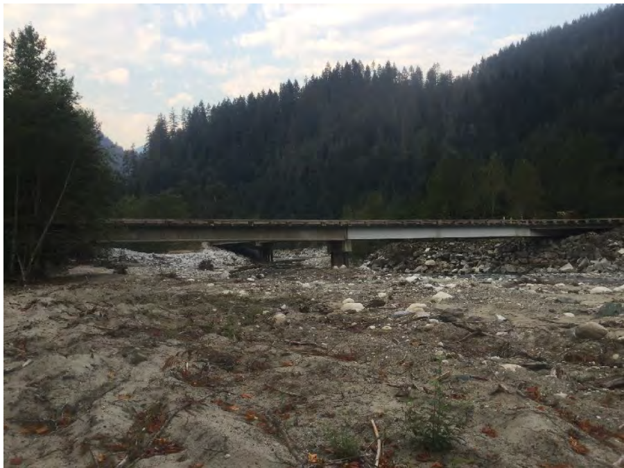
Photo 2 Bridge elevation from upstream
