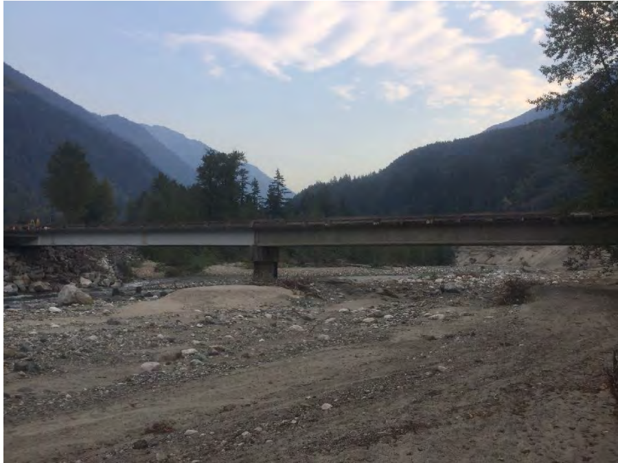
Photo 1 Bridge elevation from downstream
