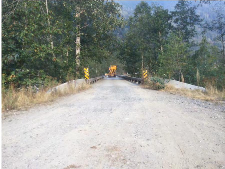
Photo 5 Left approach looking towards bridge
