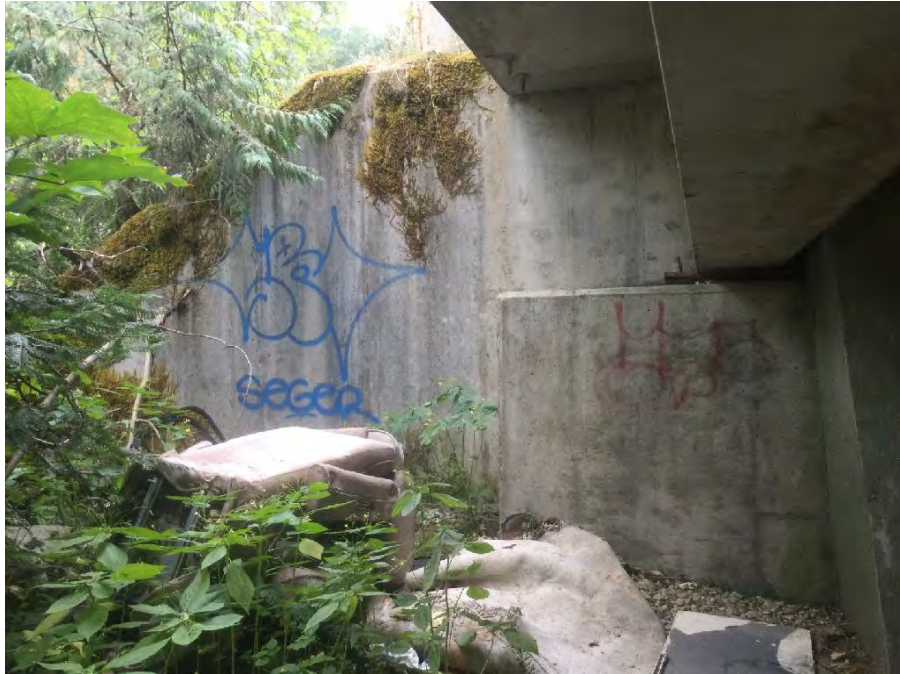
Photo 15 Left upstream wing wall
