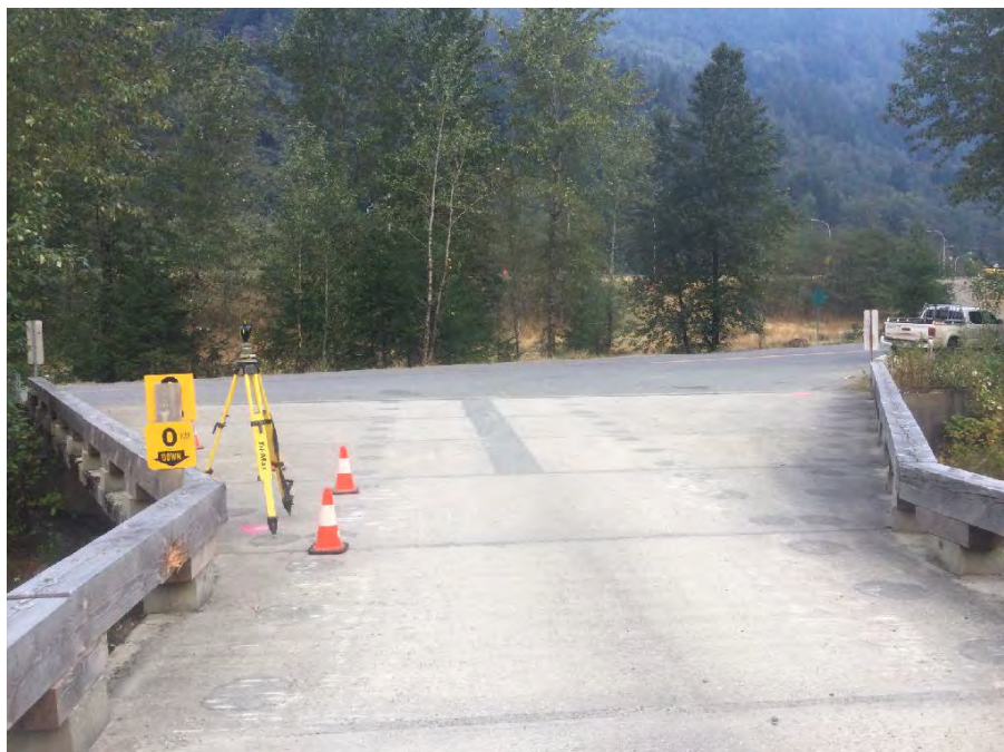
Photo 8 Right approach looking away from bridge
