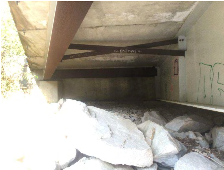
Photo 18 Right downstream wing wall
