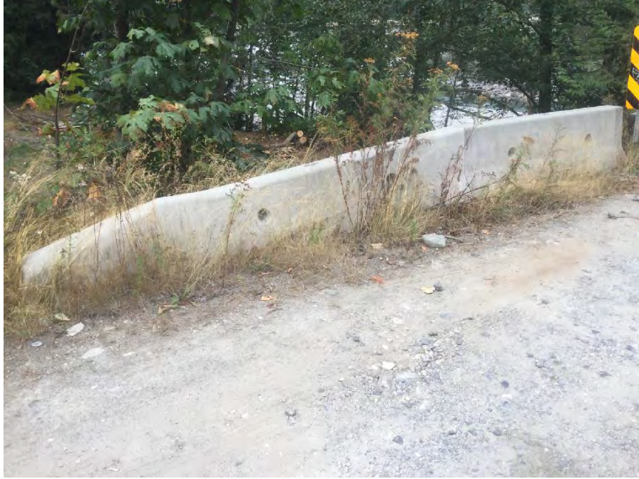
Photo 11 Typical barrier condition
